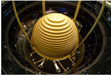
Figure 1 : Tuned mass damper
